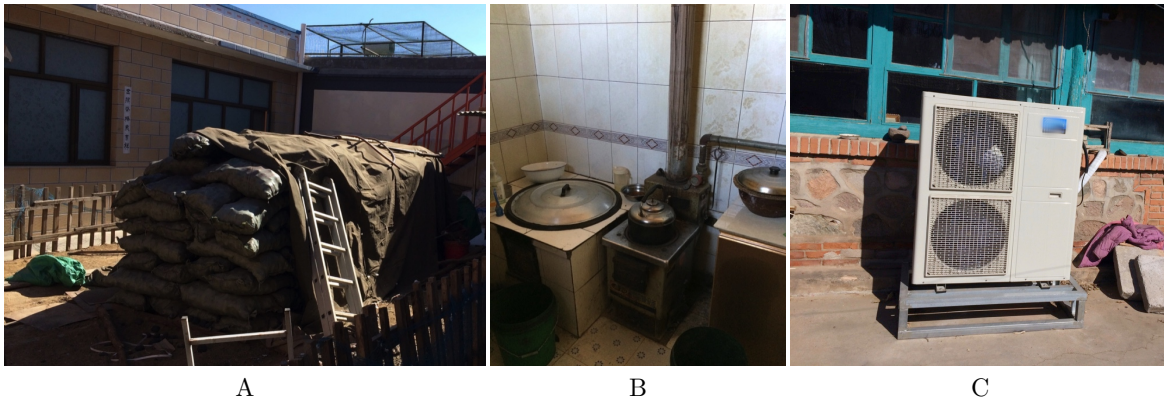
Figure 1: Coal storage and heating equipment. Coal storage for one household's winter needs is typically conspicuous (A). In (B), a cook stove to the left and a coal heating stove in the middle are both vented to the outside. The coal stove heats water for consumption as well as for distribution through radiators. In (C), a typical compressor for air-source water-heating heat-pump systems is also conspicuous outside a home in a treated village.
